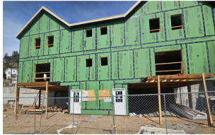
Progress on phase 2 Idaho Springs!
